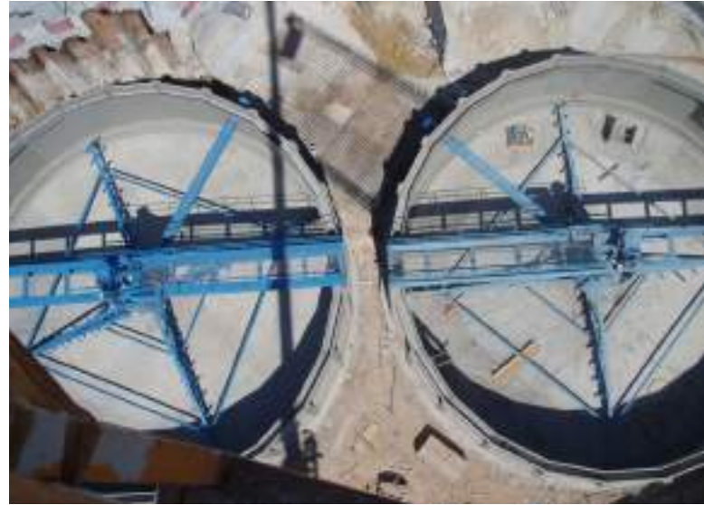
Industrial wastewater treatment plant. Flow 1.000 m 3 /h.
